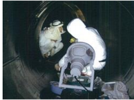
site lining (inner surface) at girth welded portion (Minimum
