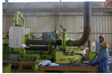
On-site bending machine
