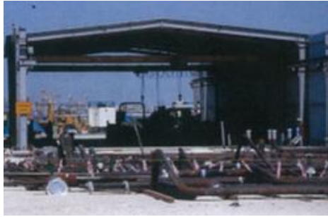
Bending machine in operation on-site
